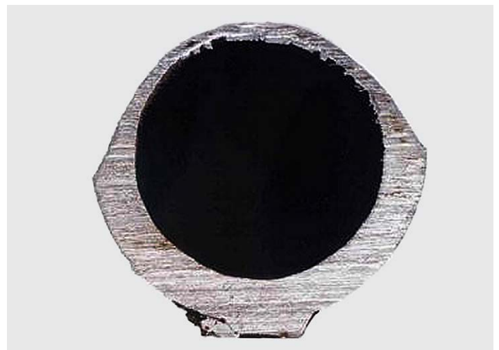
A boiler tube that has a thin wall as a result of erosive conditions.
